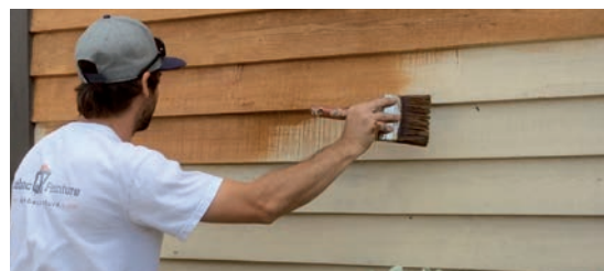
PHOTO 3 - APPLY THE 2ND COAT EQUALLY AND BRUSH TO EVEN OUT THE STAIN.
