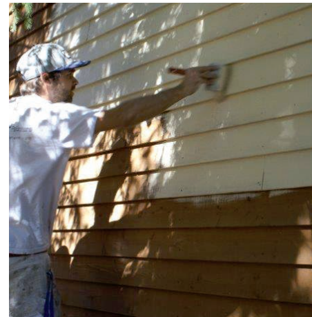
PHOTO 1 - APPLYING THE FIRST COAT (SOLID STAIN) ON HORIZONTAL SIDING.
